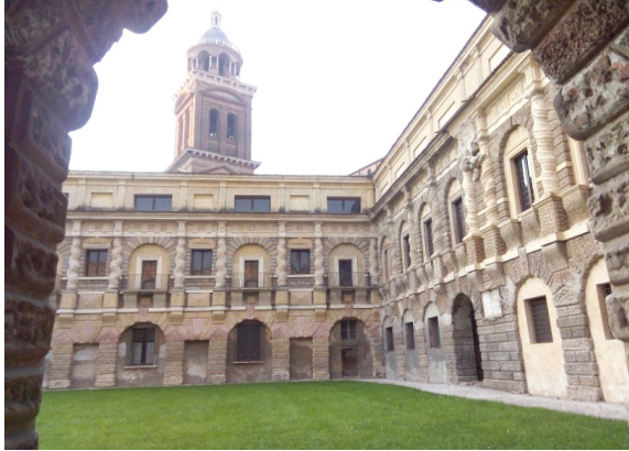
Figure 10. The courtyard of La Rustica (now Cortile della Cavallerizza ) near Palazzo Ducale
