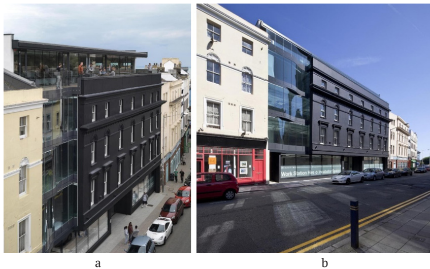
Figure 4. Reconstruction of a residential building with an extension and a superstructure
