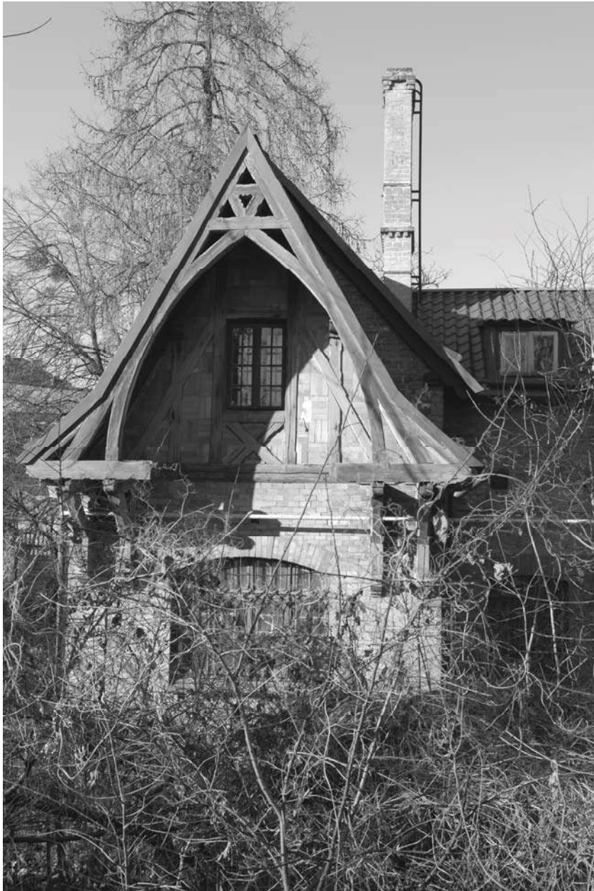
Fig. 4. The facade of the house on 14a Metrologichna St. – villa “Julietka” (photo by Yu. Bogdanova, 2019)
