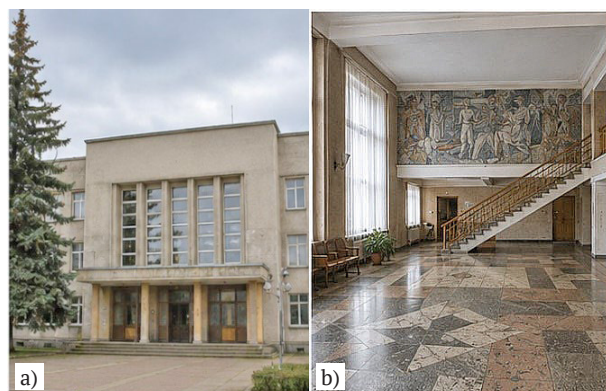
Figure 3. Stebnyk Community Centre, Stebnyk, Lviv Region
