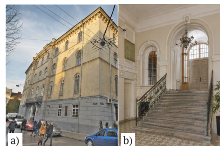
Figure 5. Zhovkva Town Community Centre, Zhovkva, Lviv Region
