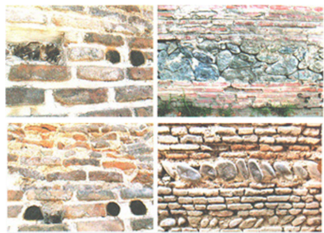
Figure 1. Stone-and-brick masonry patterns in the defensive walls of Ganja
