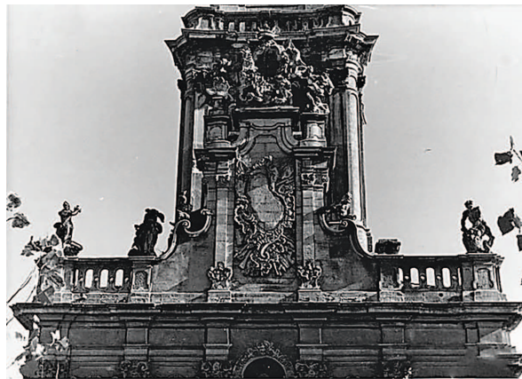
Figure 5. Pediment of the main western facade of the town hall in Buchach (archive photo)
