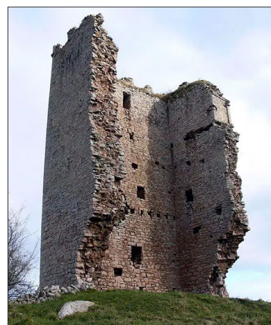
Figure 2. Photo of the Peneudes Tower
