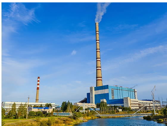
Figure 1. Ekibastuz State District Power Plant
