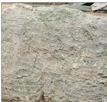
Figure 13. External surface of the wall block made of glauconitite, hewn with a flat mason's hammer
