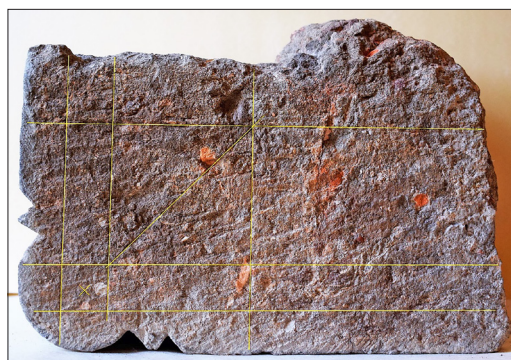
Figure 20. Marking with a spike or nail of a modular grid (guilloche) on the upper surface of a profiled glauconitite block
