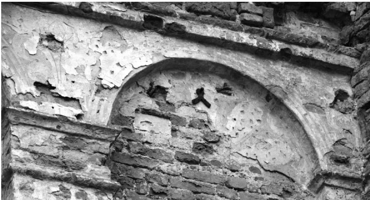
Fig. 7. Hand-drawn archivolts and half-rosettes in the arch belt on the 3rd tier of the outer wall of the tower. On the left side to the arch are fragments of a rose with branches
