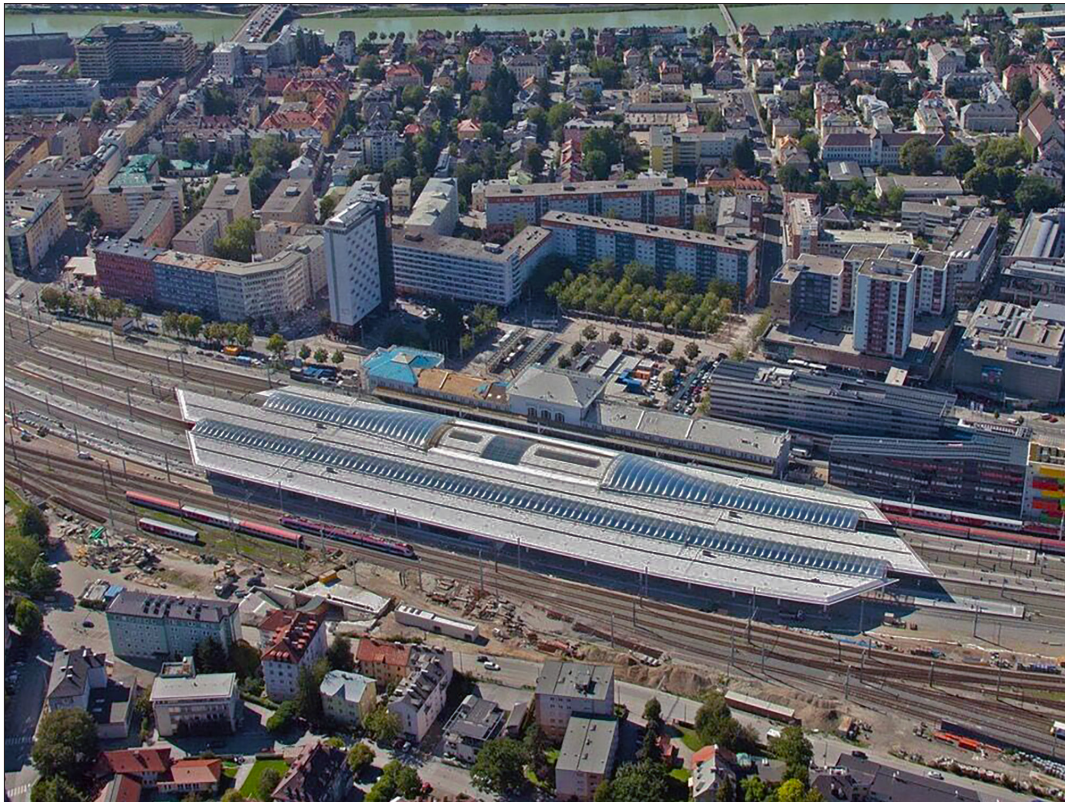
Figure 12. General view of the Salzburg Main Railway Station
