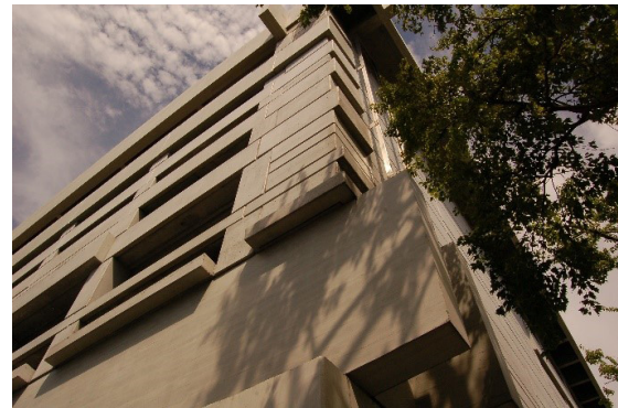
Figure 16. External corner connection on the facade of Kurashiki Town Hall
