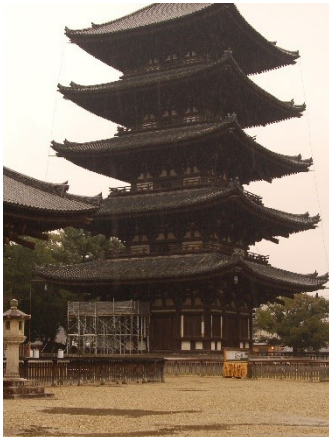
Figure 23. General view of the five-tiered pagoda of Kofukuji Monastery in Nara
