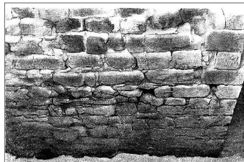
Figure 4. Photo of the North-Western part of the castle wall; excavations by P. Pokryshkin, 1912 Notes: two ways of building a wall can be easily distinguished: 1 – the lower layer is conscientiously and efficiently constructed, 2 – the upper part (the top two rows) is constructed not as carefully. There are also two types of stone blocks – a) of a clear cubic shape and b) when only the front surface and the bottom and top planes of the blocks are quilted evenly, and the two side planes have a broken irregular shape Source: P. Rappoport (1954)
