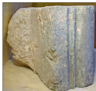
Figure 8. An example of a profiled glauconitite block “with a hook” – a protrusion in the rear inner part for better binding and “hooking” the block in the wall Source: photo by M. Bevez
