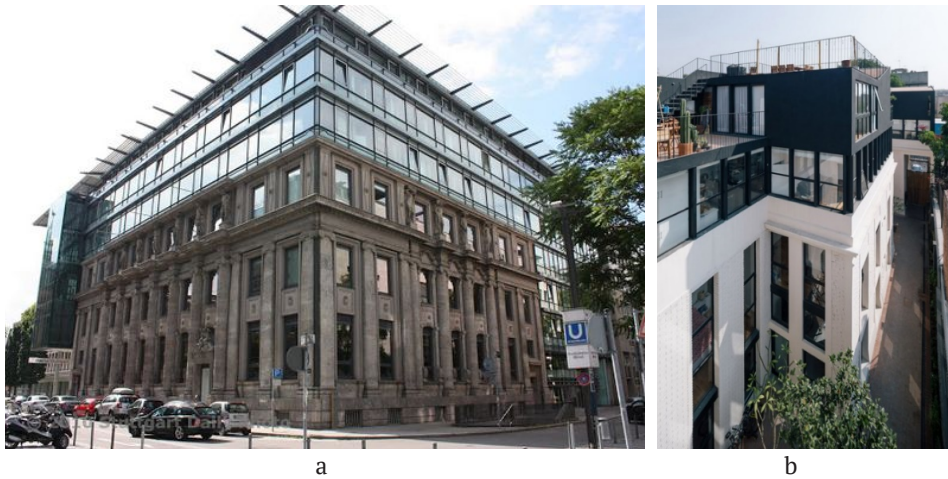
Figure 3. Reconstruction with a superstructure
