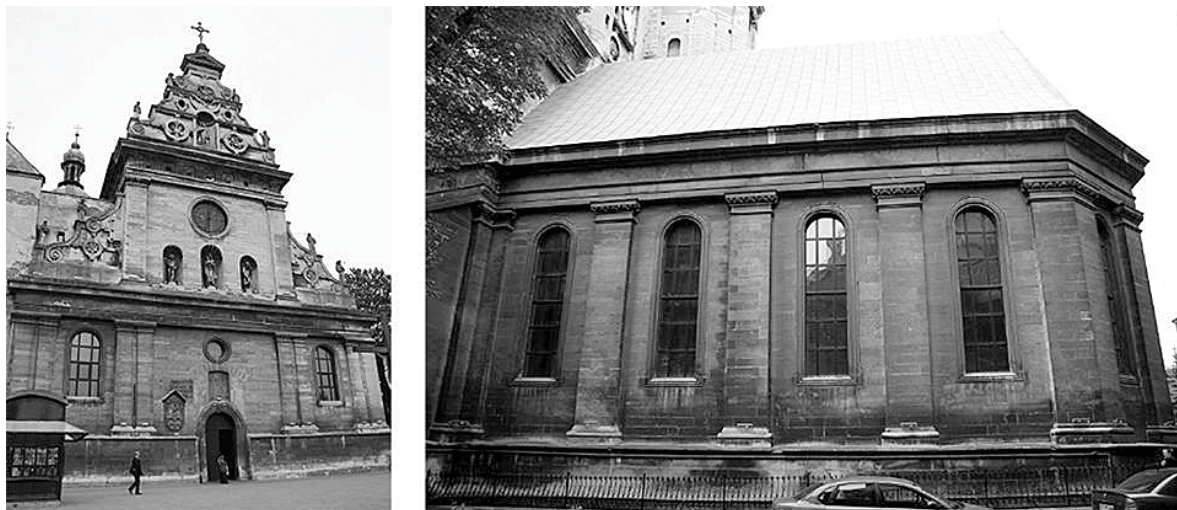
Fig. 13. P. Dominici, St. Andrew Church, photography, Lviv, built from 1600 (left) P. Dominici, St. Andrew Church, view from the south, photography, Lviv, built from 1600 (right) Source: S. Husak, 2016
