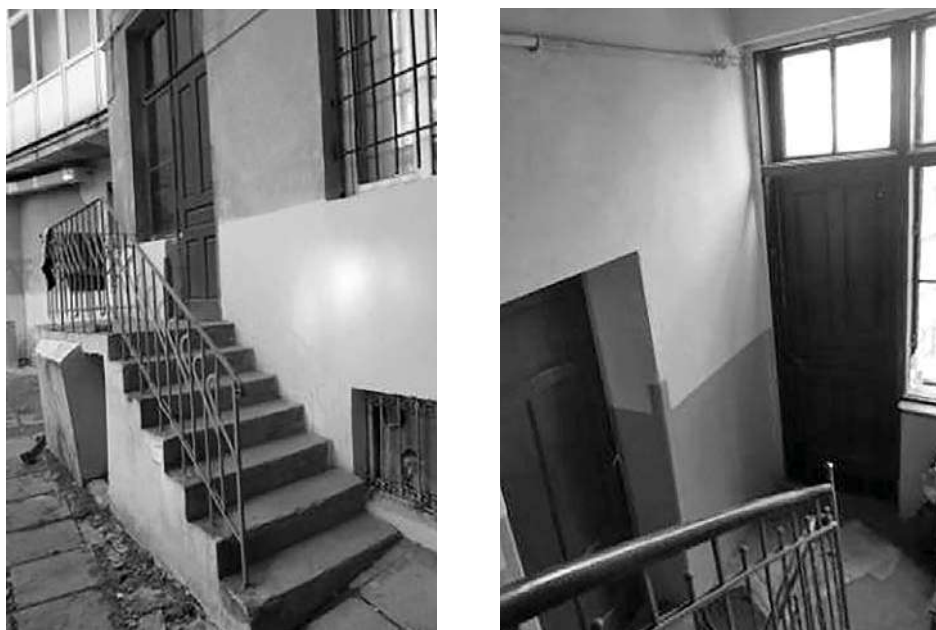
Fig. 8. Entrance to the black staircase of house No. 14 from the common yard with house No. 16 on Kost Levitsky street and a fragment of its interior
