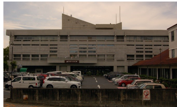
Figure 17. Exterior of the Kurashiki Town Hall
