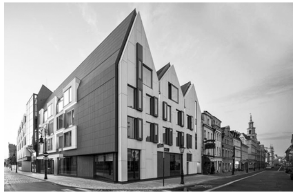
Fig. 6. A new accent angle fixation in the historical environment. Poznan, Poland. Photo [12]
