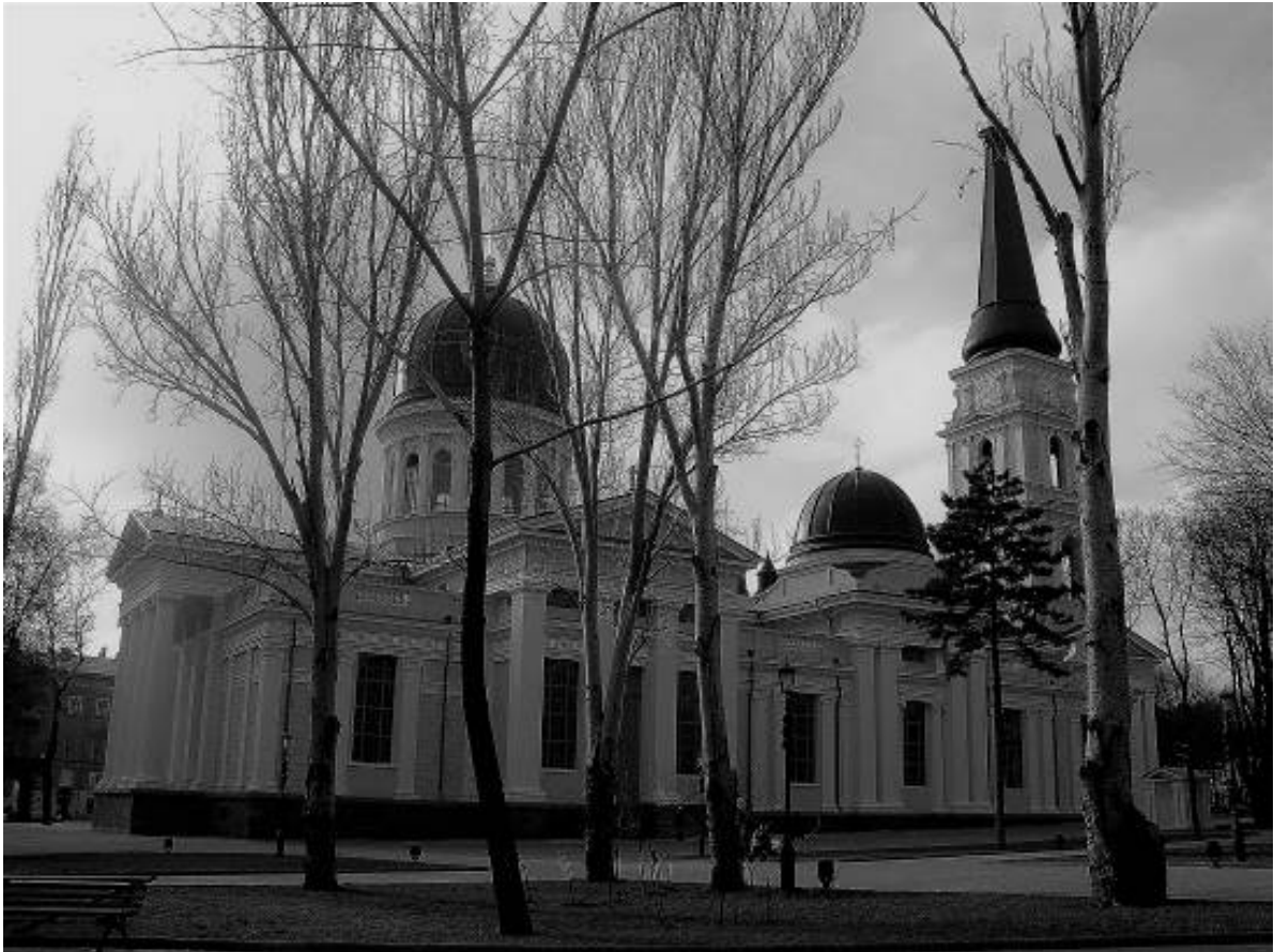
Fig. 9. Reconstructed Transfiguration Cathedral in Odessa. Source: The V. Meshcheriakov archive
