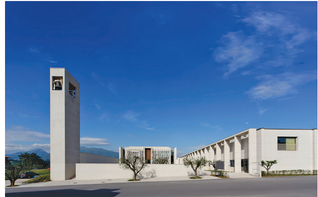
Figure 11. Church and Community Centre in Castel di Lama
