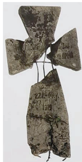
Figure 5. Reinforced concrete cross rifleman of the Ukrainian Galician Army from the city of Belza before the conservation
