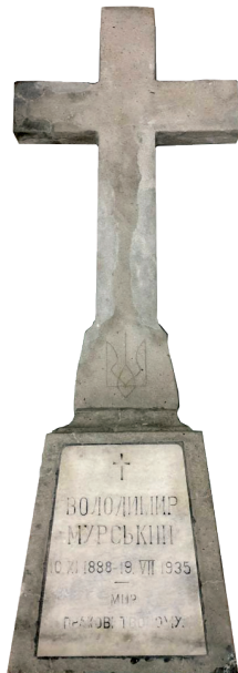
Figure 2. Reinforced concrete tombstone cross of the Volodymyr Murskyiv after restoration
