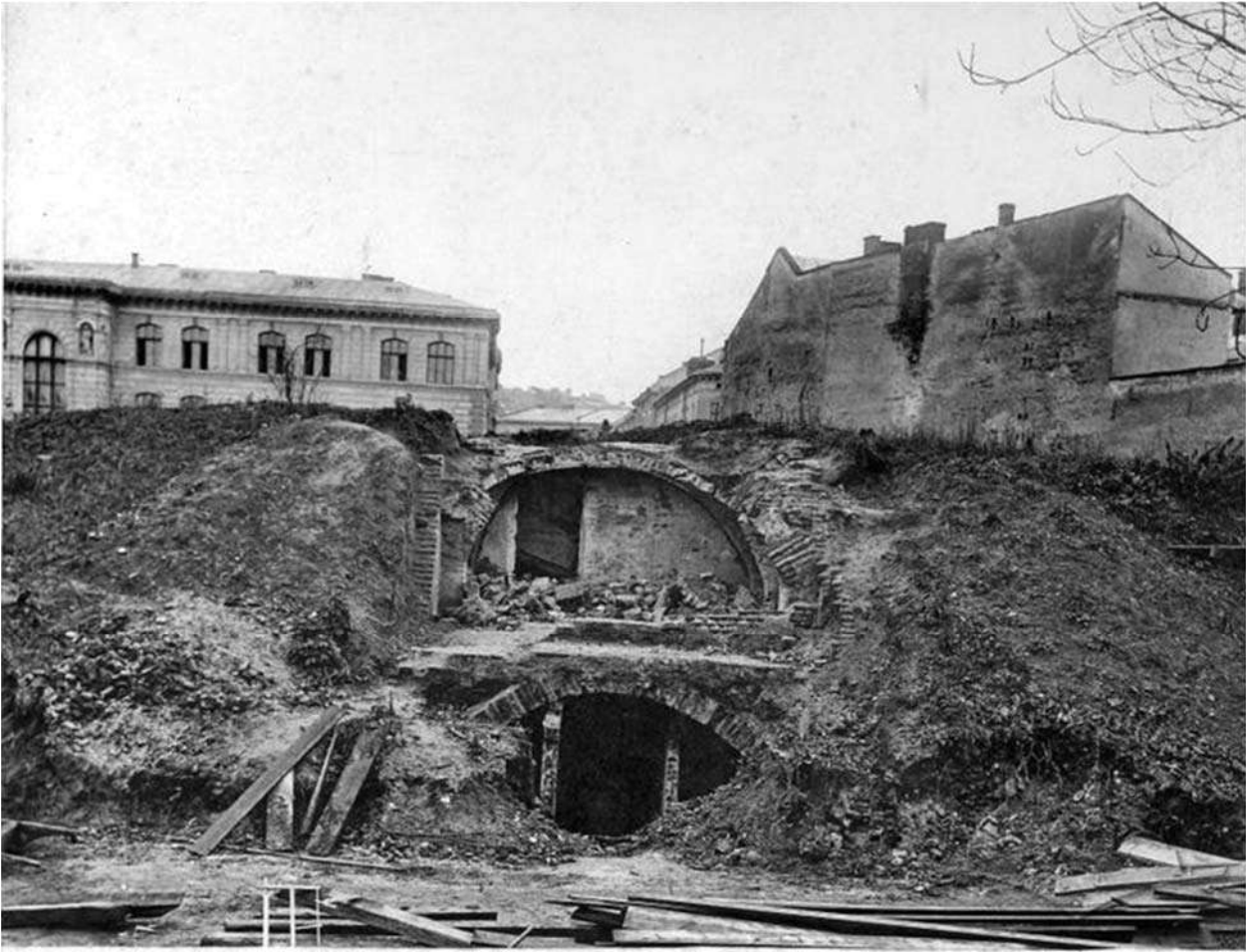
Fig. 15. Photo of the dismantling of the southwestern bastion of the Behrens line, the 1890s, photographer Marek Munz (Lviv, 2006). From the photo, it can be seen that the height of the bastion reached 11–12 m
