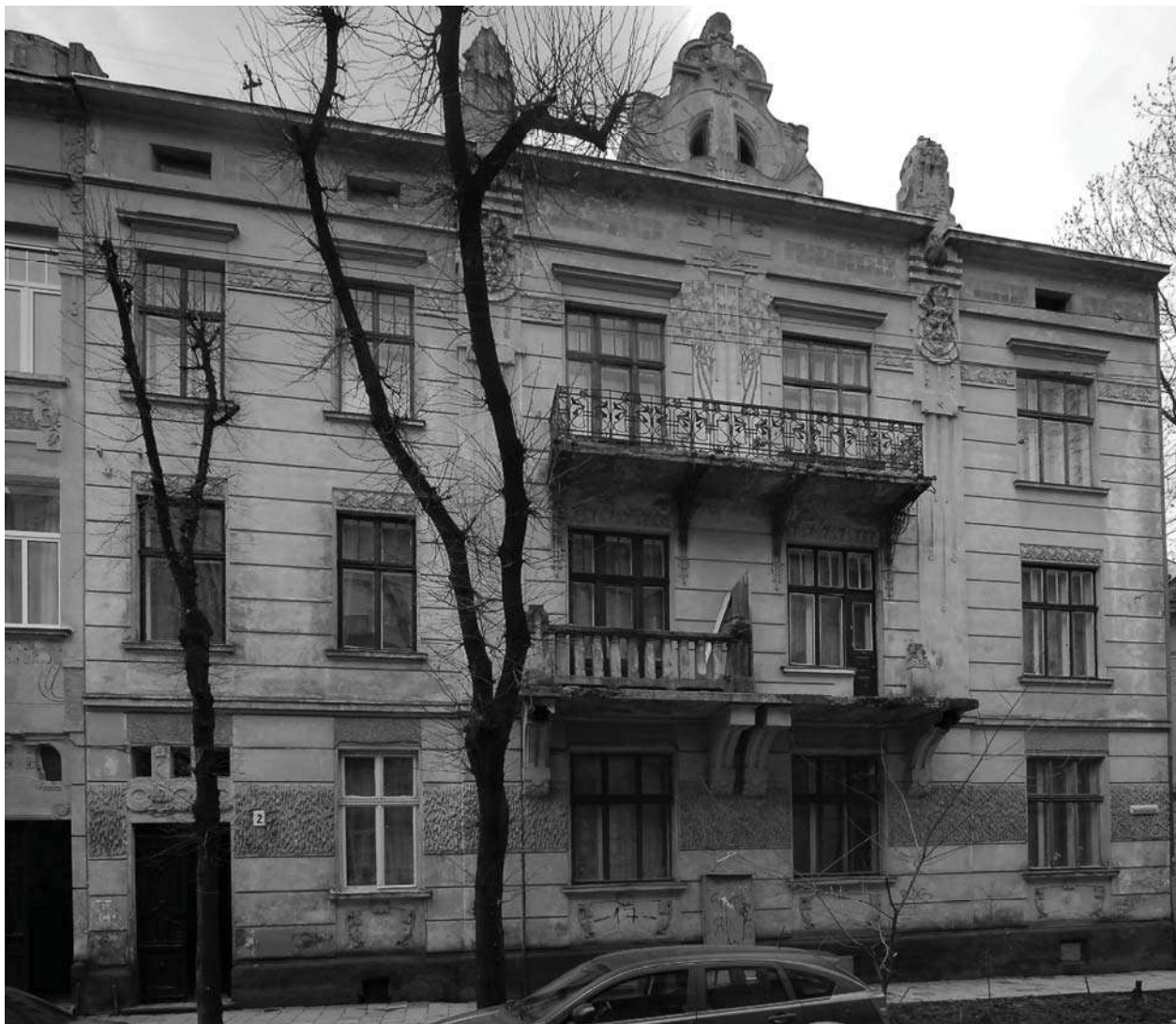
Fig. 3. Residential house, 2 Akademik Pavlov Street, 1905–1906. I. Levynsky's office (Foto Yu. Bohdanova)
