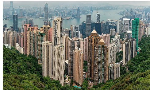
Figure 2. Panorama of high-rise residential buildings in Hong Kong
