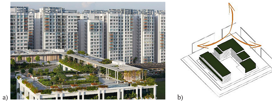
Figure 2. Innovative approach to urban landscaping in the context of an extensive principle of its implementation
