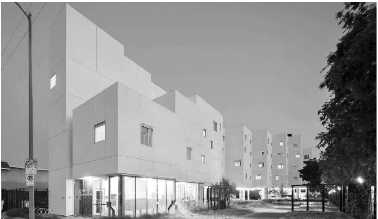
Fig. 6. Modern homeless facility in Los Angeles, USA
