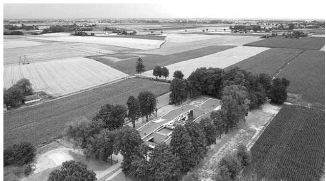
Fig. 5. A housing and industrial rehabilitation complex for the homeless in Krakow, Poland
