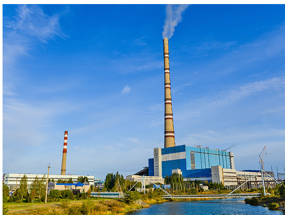
Figure 1. Ekibastuz State District Power Plant
