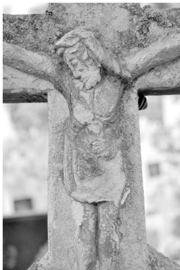
Fig. 9. An example of damage caused by unprofessional painting of limestone
