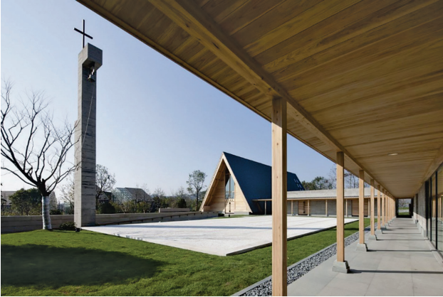
Figure 1. Mei Li Zhou church. Tsushima Design Studio Source: based on Mei Li Zhou Church/Tsushima Design Studio (2010)
