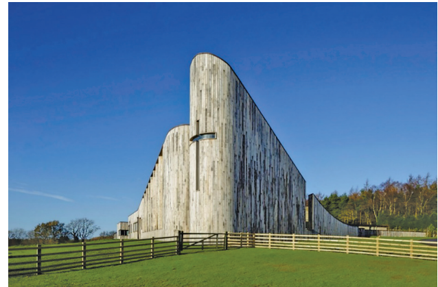
Figure 4. Stanbruck Abbey complex in United Kingdom Source: based on Stanbrook Abbey/Feilden Clegg Bradley Studios (2015)
