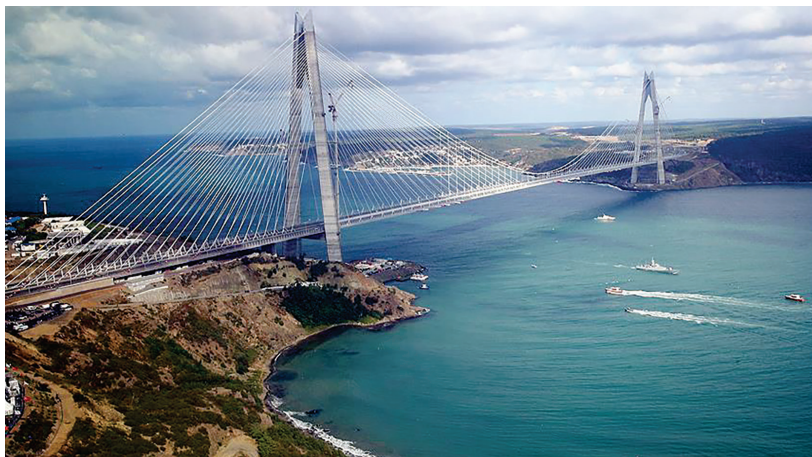
Figure 2. Bosphorus Bridge (Turkey)
