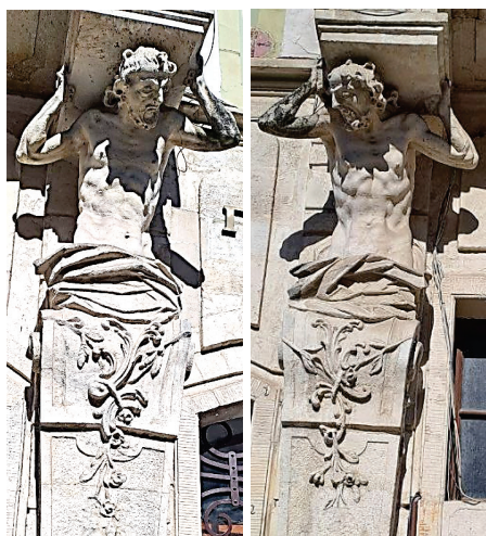
Figure 9. Consoles in the form of male torsos of house No. 40 on Rynok Square in Lviv Source: authors' photo (2024)
