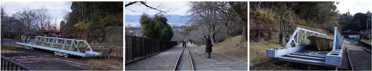
Figure 2. Keage Incline and rail platforms between the upper and lower distribution ponds
