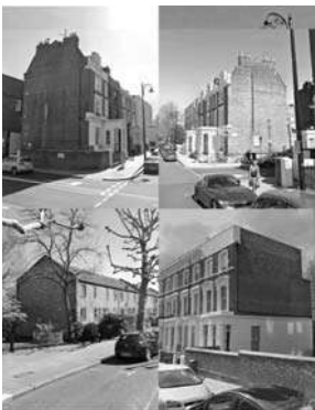
Fig. 1. Unused blank facades in London [Google Earth]
