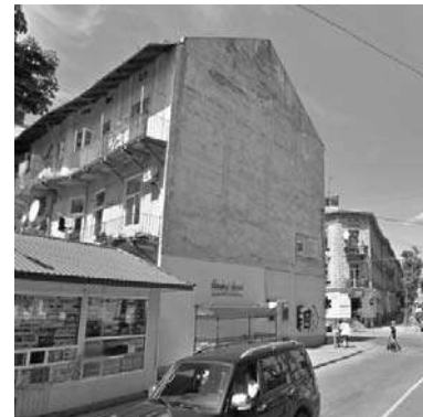
Fig. 3. Huge blank façade in Lviv [Google Earth]
